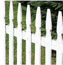
Fences and Walls
