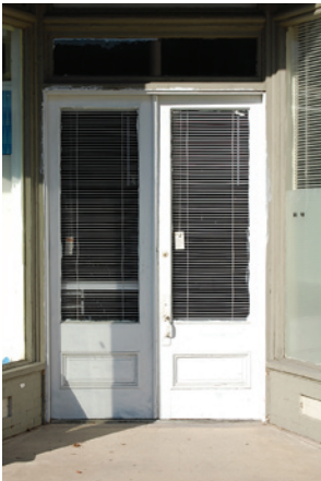
Storefronts typically see a lot of change. Surviving wood doors are rare and should be kept and preserved.
