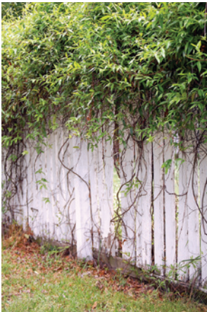
Climbing vines make maintenance more difficult and can weaken a fence or throw it out of alignment.
