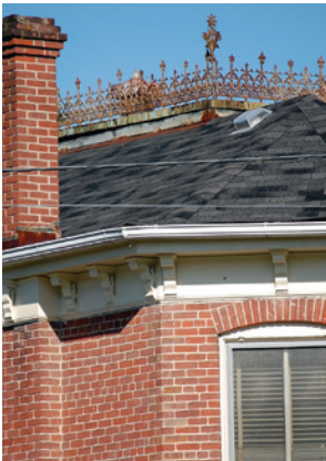
Cresting, which is ornamental work at a roof ridge, is not a common architectural detail in Franklin. An excellent example can be seen on this Italianate house on High Street.
