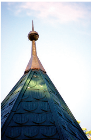
Finials, on the other hand, are not at all unusual in the residential section of Franklin's Historic District. Finials are roof ornaments most often seen at the peak of a conical or pyramidal roof. Several Queen Anne dwellings in Franklin feature finials.
